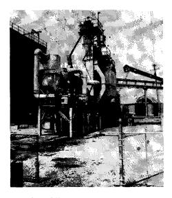
• French Oil Mill Machinery has installed two new stationary louver meal/dryer coolers at Plains Cooperative Oil Mill in Lubbock. The modular stack-type design units can be added to existing French cookers. Units are available in capacities from 25,000 to 100,000 pounds per hour. Information: Solvent Extraction Division, The French Oil Mill Machinery Co., Piqua, OH.
